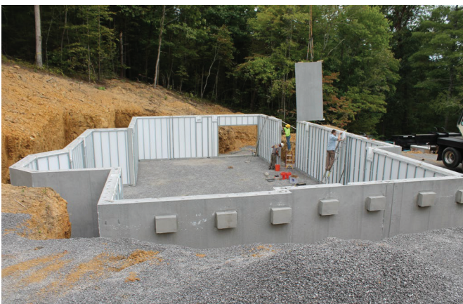
Completed Basement Ready for the Floor System
