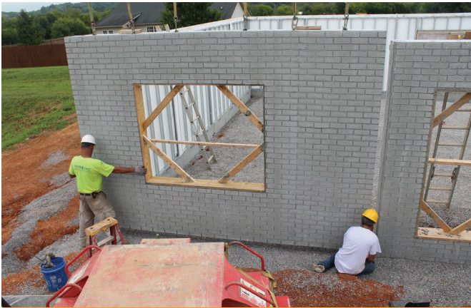
Installation of Above Grade Walls
