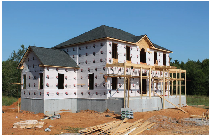
Residential Basement Framed Out
