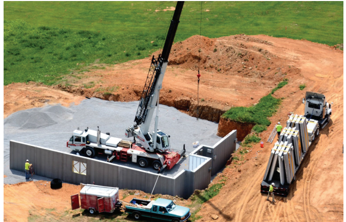
Residential Basement Wall Installation
